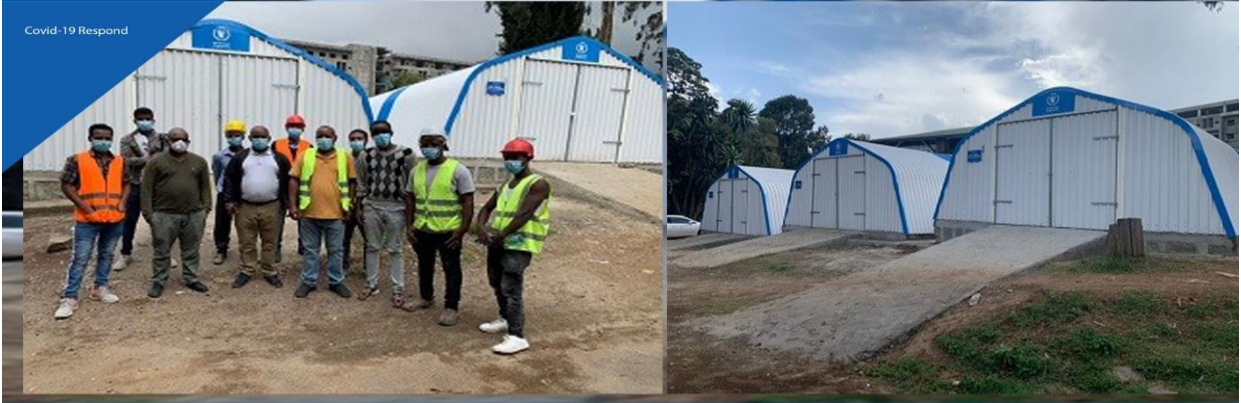
Flowspan construction to support Ethiopian Public Health Institute Support (EPHI)
